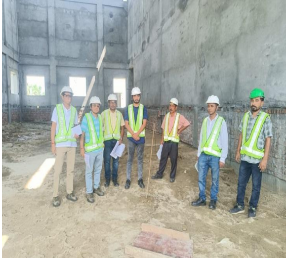
Photo Plate 1 – Site visit by PMC officials at Burhigaon substation.
