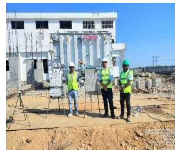
Photo Plate 28 – Post-monsoon EQM conducted at Nagaon-2 S/S.
