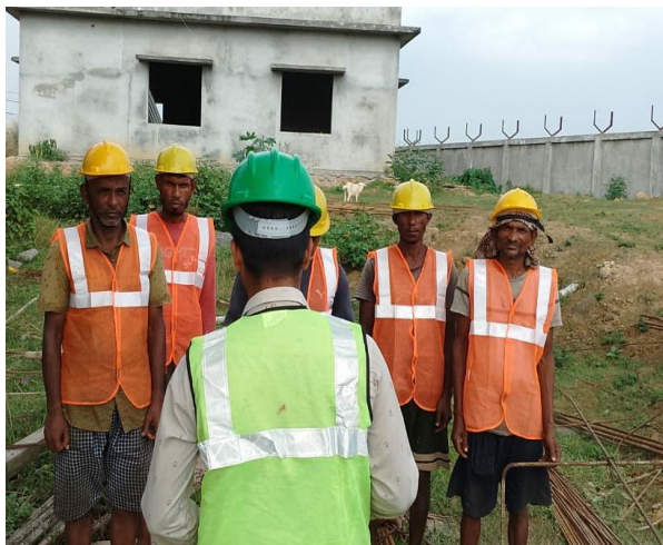
Photo Plate 17 – TBT conducted regular basis at Jakhalabandha S/S
