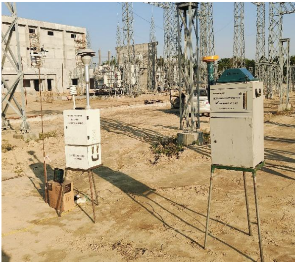
Photo Plate 23 – EQM (Air) at Sonapur S/S.
