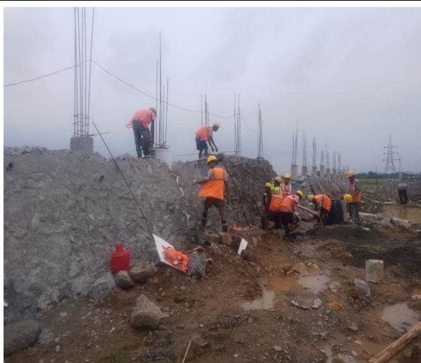
Photo Plate 15 – Workers were working with full equip with PPEs at Sonapur S/S.
