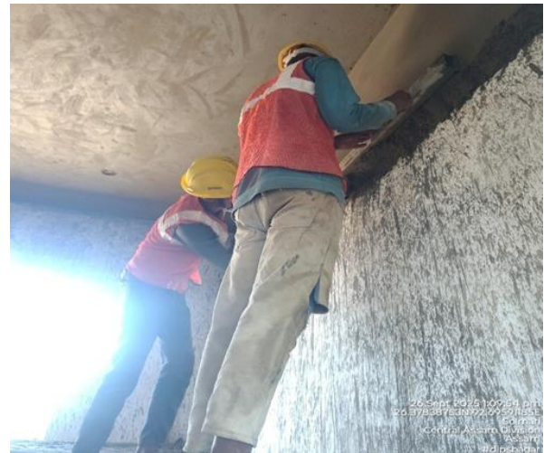
Photo Plate 18 – Workers were fully equipped with PPE at Nagaon-2 S/S
