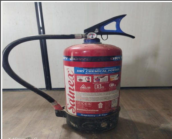
Photo Plate 43 – Fire extinguisher provided to labour camp at Khumtai Substation
