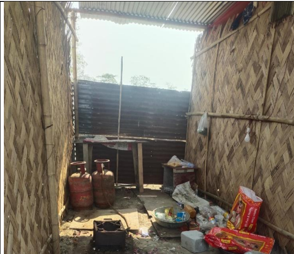
Photo Plate 7 – LPG cylinder provided in the labour camp at Khumtai S/S
