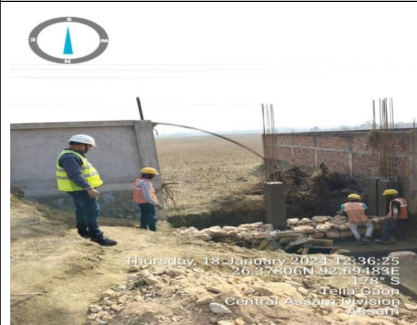
Photo Plate 3 – Workers are well equipped with PPE at Nagaon S/S
