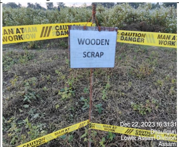
Photo Plate 11 – Barricading done around the Agomani substation area.
