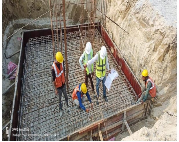
Photo Plate 20 – Workers are well equipped with PPE at Agomani S/S
