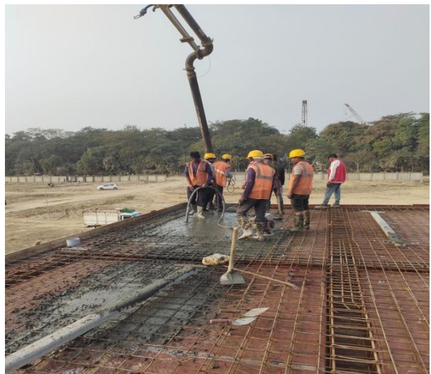
Photo Plate 16 – Working working with PPEs at Khumtai S/S
