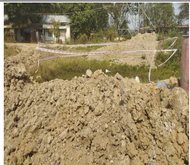
Photo Plate 17 – Excavate pits are barricaded at Sankardevnagar S/S
