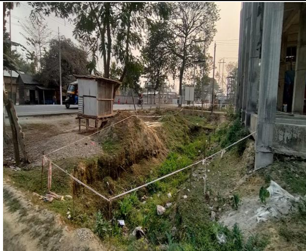
Photo Plate 13 – Barricading done at Burhigaon Substation
