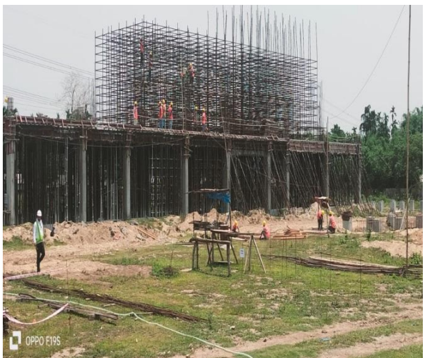
Photo Plate 46 – Workers are well equipped with PPEs at Agomani S/S
