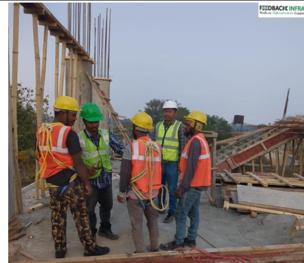
Photo Plate 3- EHS&S training program at Jakhalabandha S/S.
