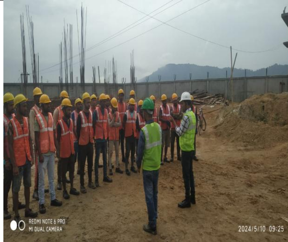
Photo Plate 7- EHS&S training program at Jakhalabandha S/S.
