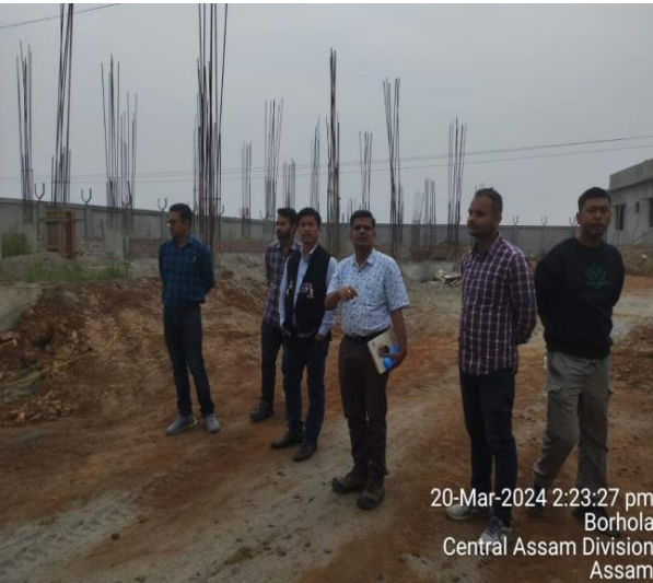
Photo plate 21 – Jointly site visit by AEGCL, PMC and EPC contractor at Jakkhalabandha S/S
