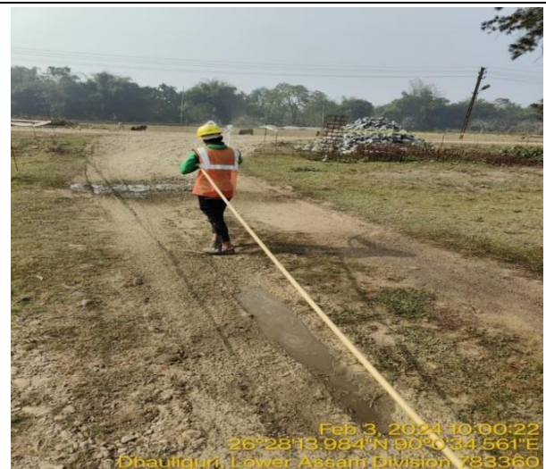
Photo Plate 18 – Water sprinkle done around the Agomani site to suppress dust.
