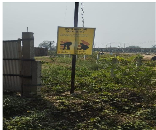
Photo Plate 10 – Caution sign placed at Sankardevnagar substation.
