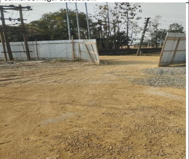
Photo Plate 12 – Housekeeping done around the Jakhalabandha S/S
