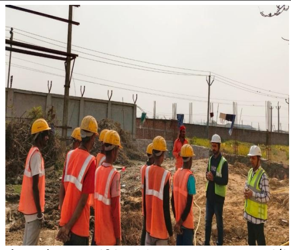
Photo Plate 4- EHS&S training program at Nagaon S/S.
