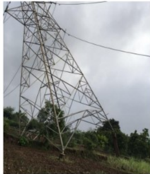
Failed tower at location no. 8
