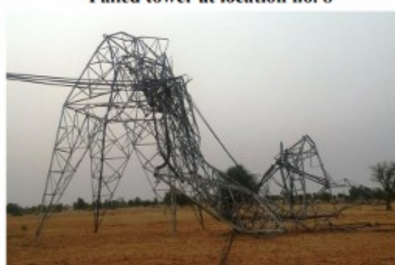
Failed tower at location no. 8
