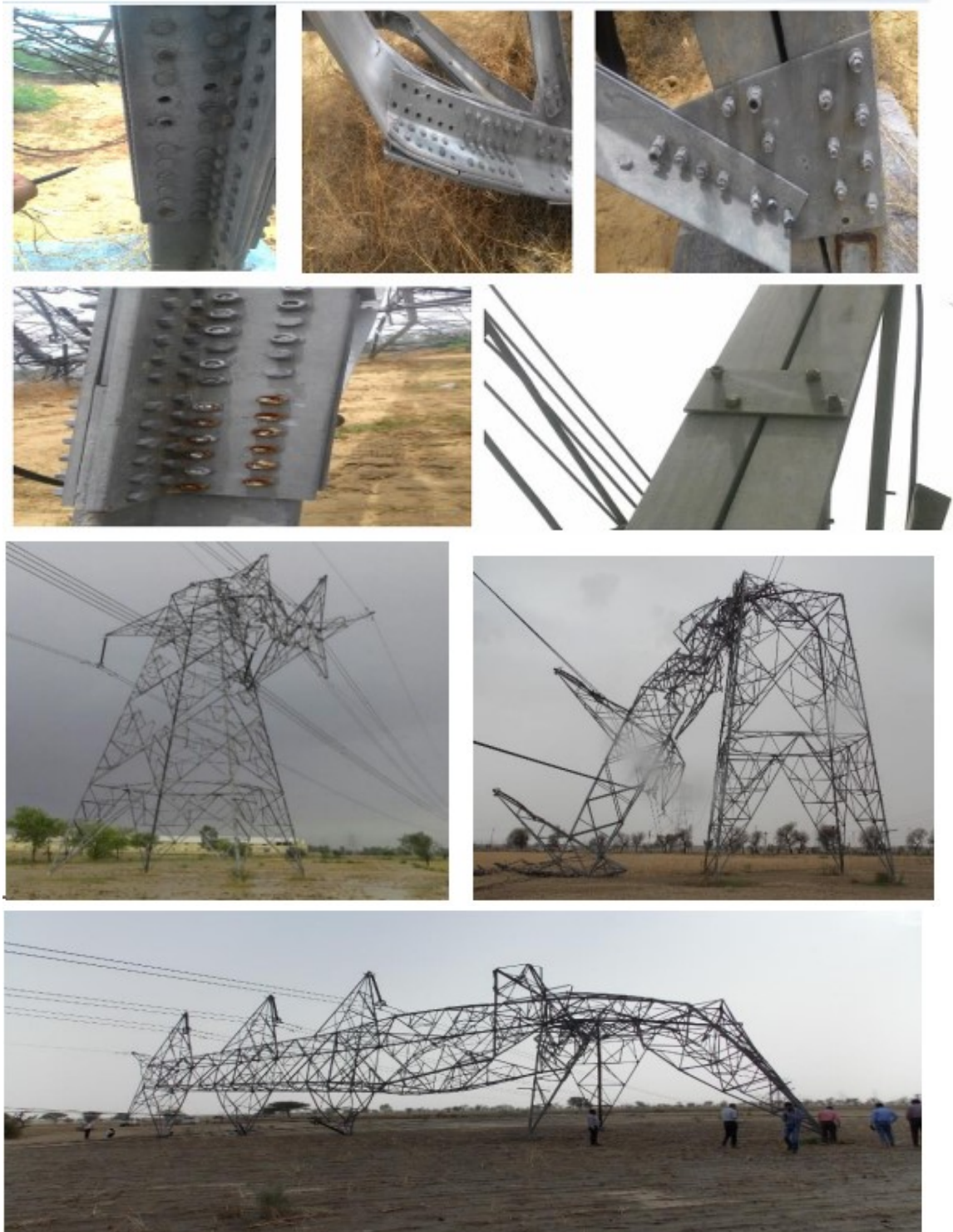
Photo Plate- Tower Collapse due to wind storm
