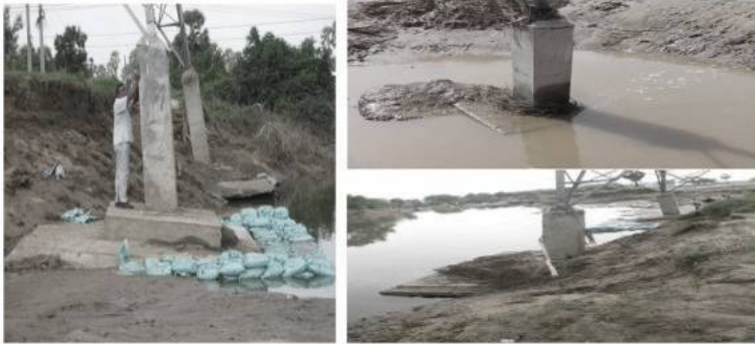
400KV D/C (QUAD) Nellore -Tiruvalem Transmission line failed on 04.12.2015 (One tower loc no.13)
