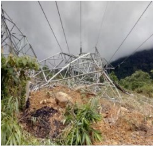
Failure of tower at location no. 56
