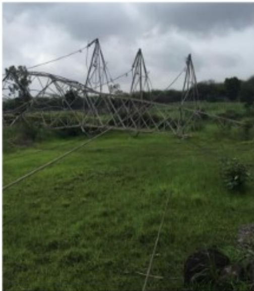
Failed tower at location no. 7
