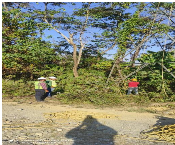
Photo Plate 35 – Earthwire dismantle and breaker recovery work in progress at Gosaigaon-Dahaligaon line (Pkg-M)
