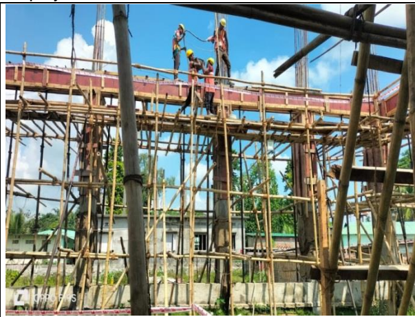
Photo Plate 22 - Workers are well equipped with PPE during GIS building beam casting work at Burhigaon S/S.
