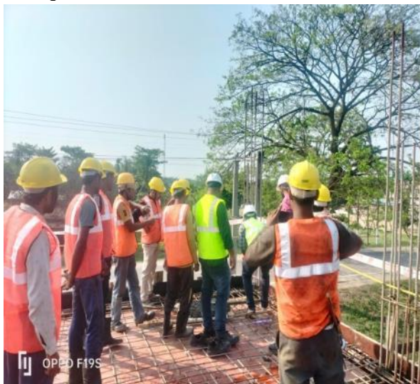
Photo Plate 9 – Workers wearing proper PPEs during slab casting work at Burhigaon S/S
