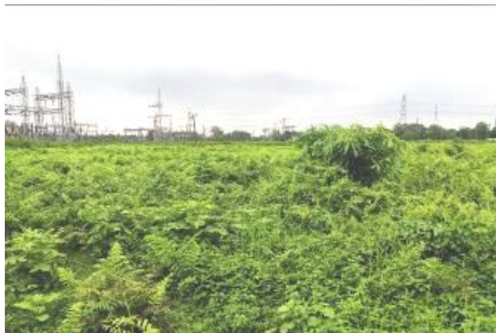
Photo plate 20: Proposed substation site
