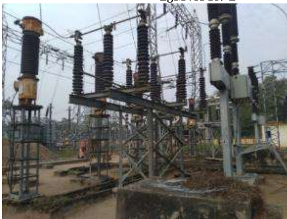
132kV Tr Breaker with CT
