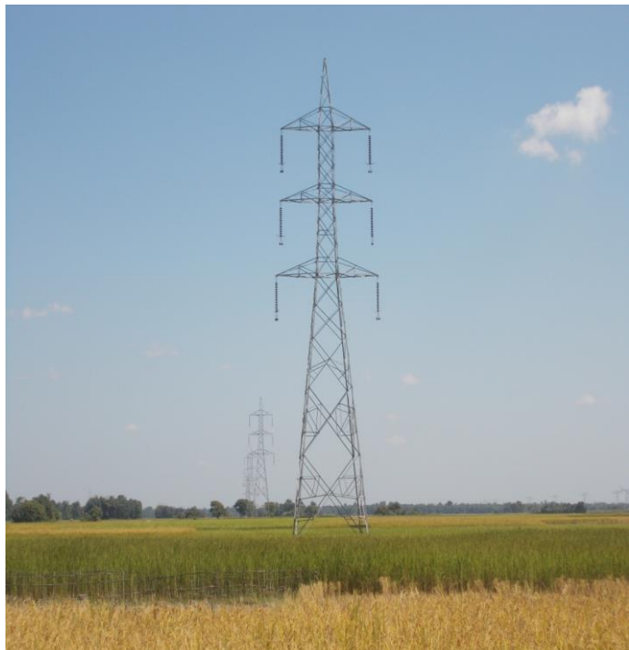
Photo 21: Completed tower erection which are passes through paddy field of 220kV BTPS T/L
