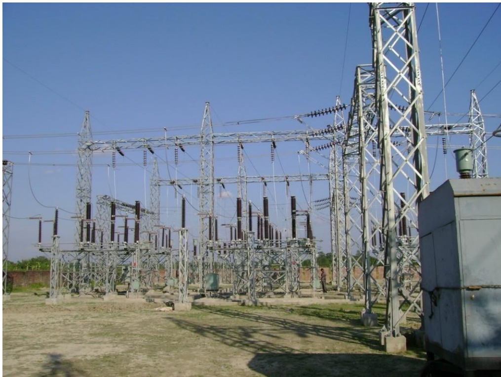
Photo 5: New 132/33 kV 2x16 MVA Substation at Nalbari
