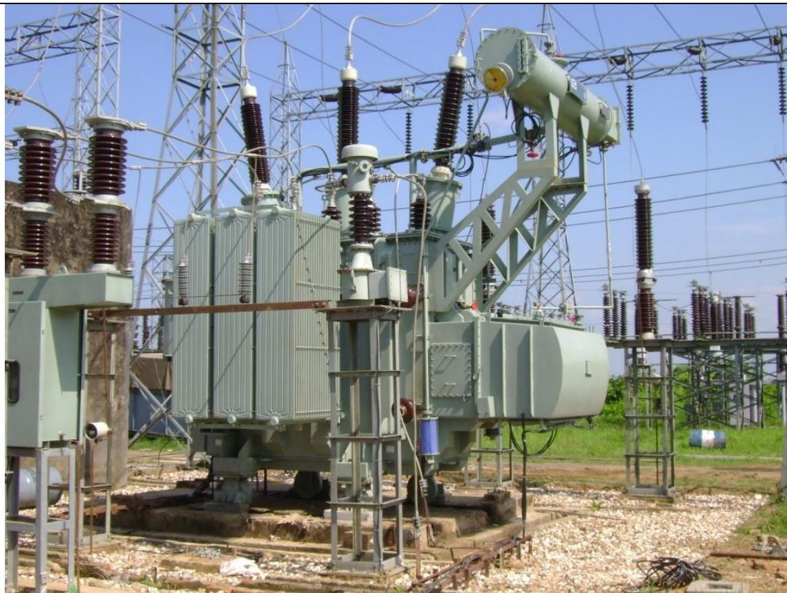
Photo 1: Commissioned 16 MVA 132/33 kV Transformer at Agia Substation
