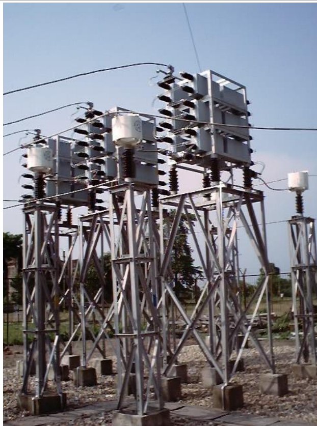
Photo 4: Commissioned 5 MVAR 33 kV Bus
