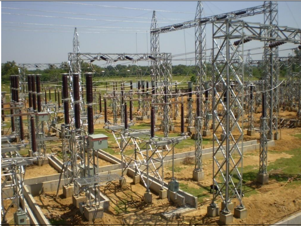
Photo 2: New 132/33 kV 2x16 MVA Substation at Boko
