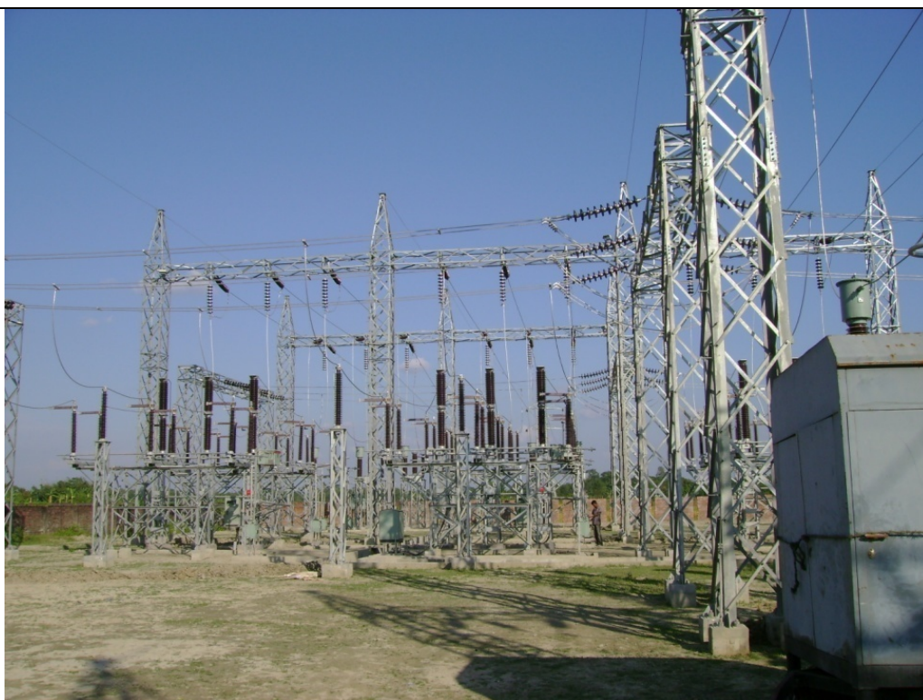
Photo 5: New 132/33 kV 2x16 MVA Substation at Nalbari
