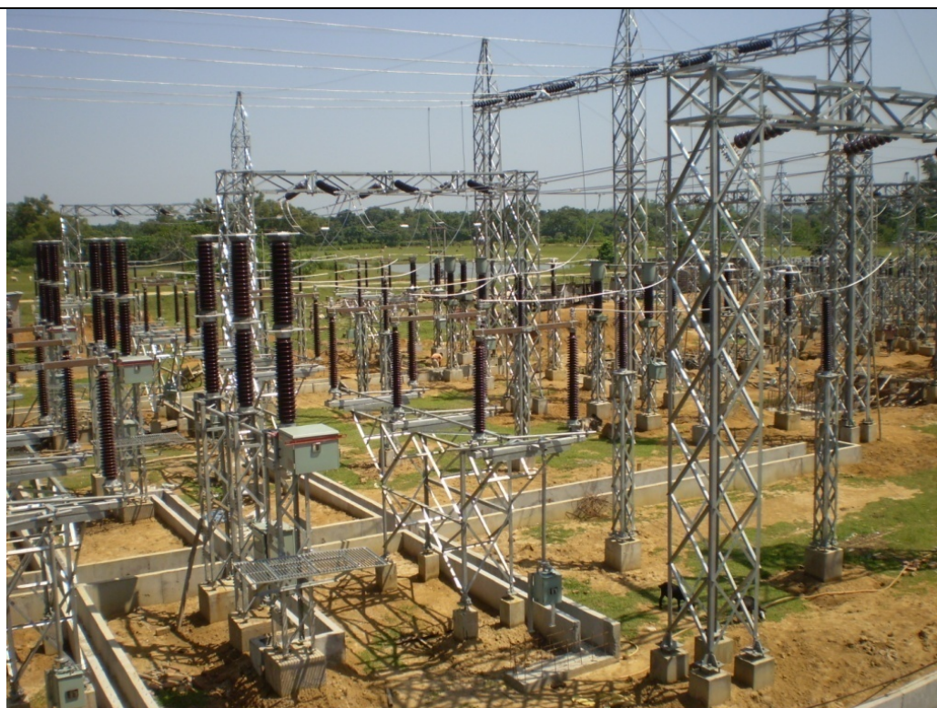
Photo 2: New 132/33 kV 2x16 MVA Substation at Boko
