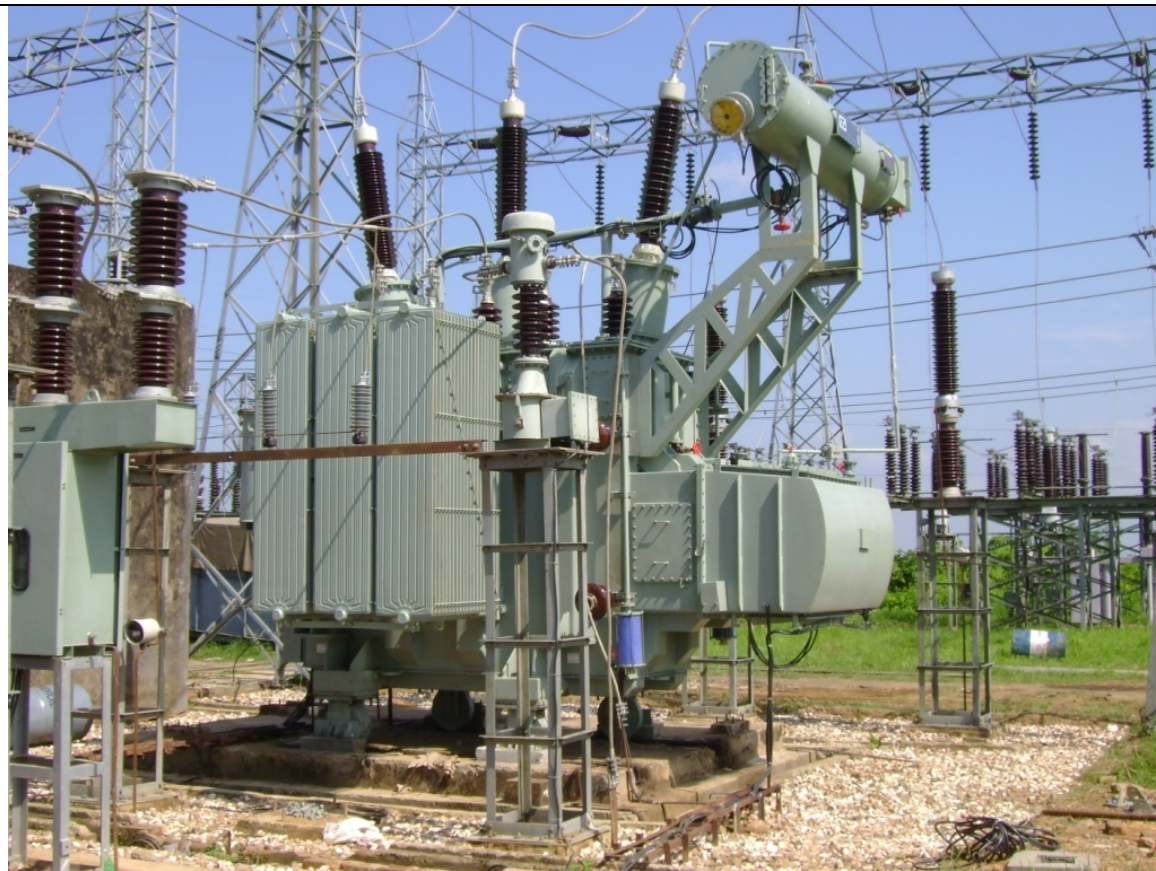
Photo 1: Commissioned 16 MVA 132/33 kV Transformer at Agia Substation
