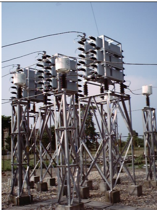
Photo 4: Commissioned 5 MVAR 33 kV Bus
